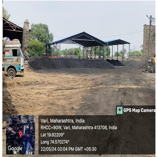
Covered coal storage shed.
